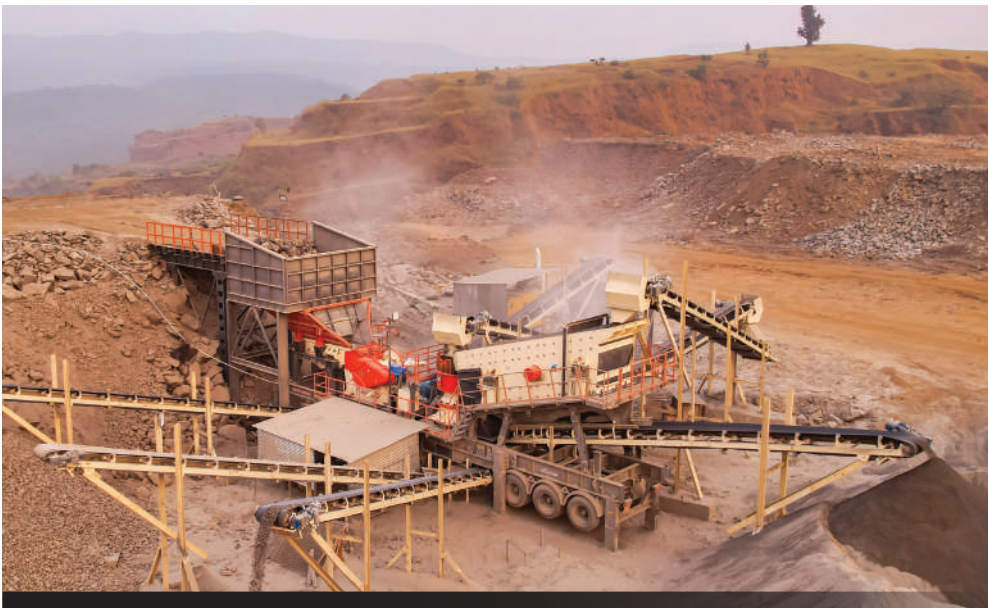
SMART 200 TPH - 2 STAGE C&S PLANT
