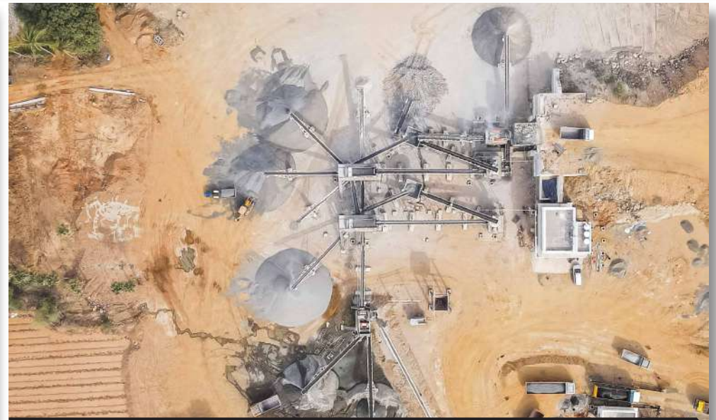
350 TPH - 3 STAGE C&S PLANT WITH WASHING SYSTEM
